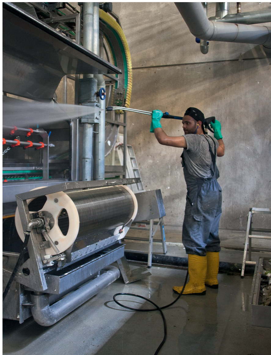
Washing plant for returnable carriers
